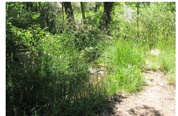
Photo 3. Overgrown conditions at Las Cuevas Ditch
