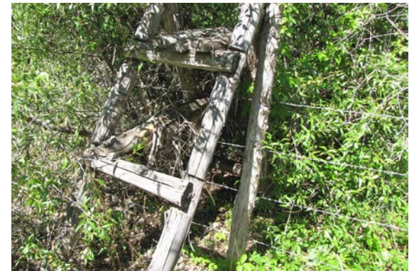
Photo 8. Existing stile, overgrown vegetation along Rio Santa Cruz
